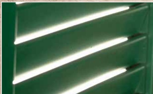
DETTAGLIO ANTA CON LAMELLE APERTE.
